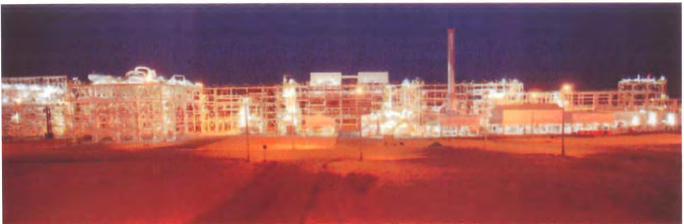
Petrofac will undertake the EPC of the gas compression system and associated facilities at the Kauther gas plant (pictured) in Oman for PDO.
